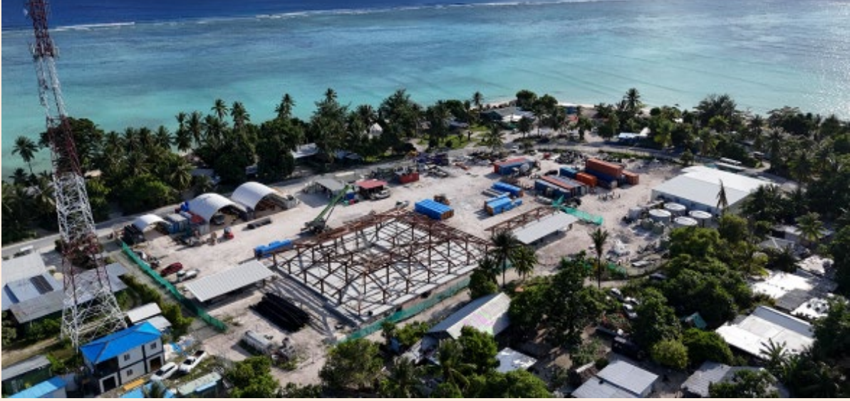
Construction of Betio Hospital, Kiribati. Credit: Reeves International
