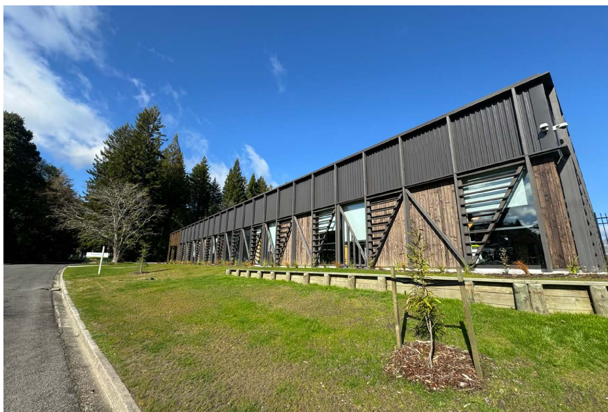
MPI's Rotorua office, a new building opened on 7 June 2024 and co-tenanted with the Department of Conservation, showcases wood construction and wool carpet tiles.
