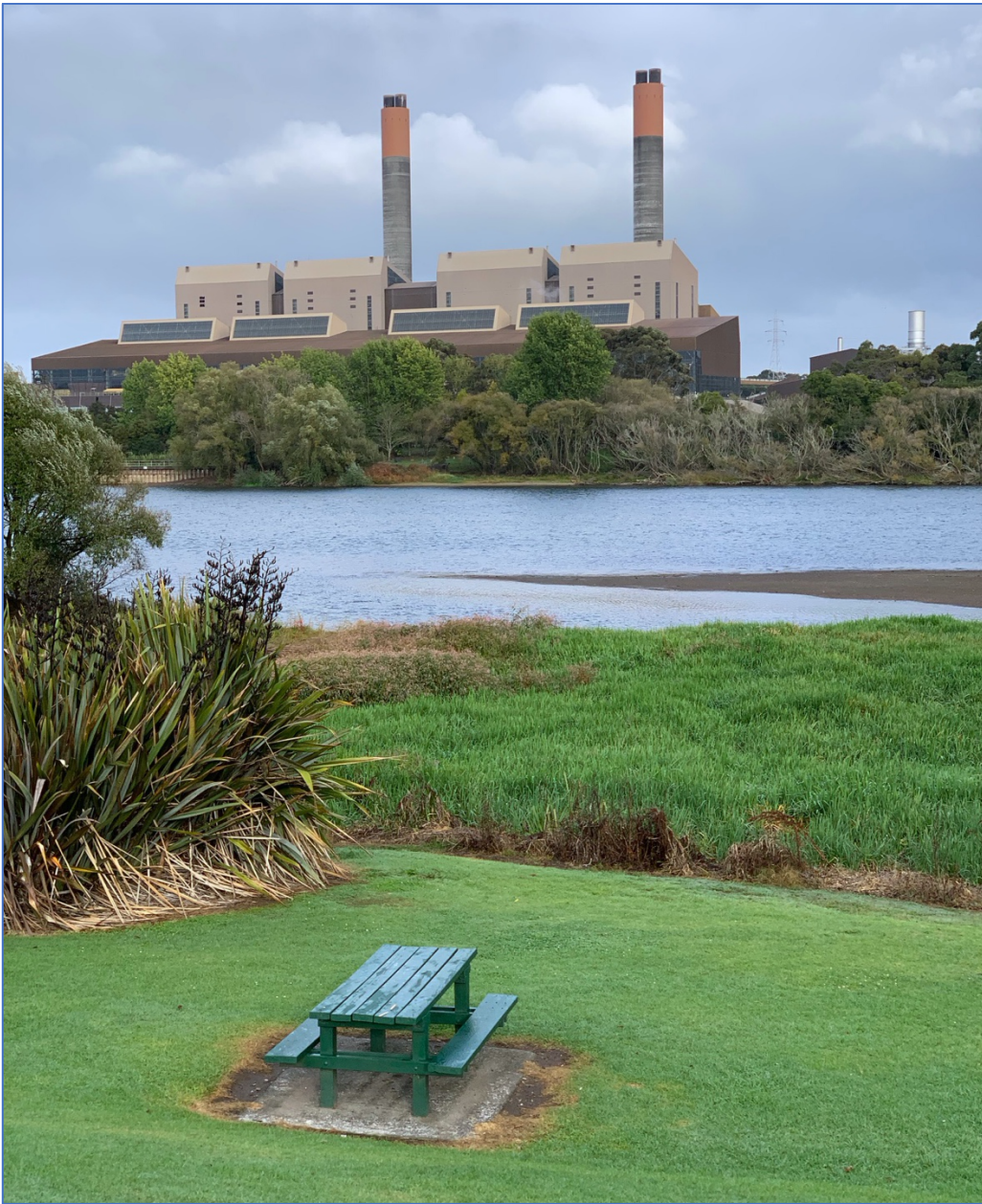
Huntley Power Station, Huntley.
