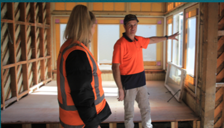
The demolition of the former Masterton hospital, showing salvage efforts
