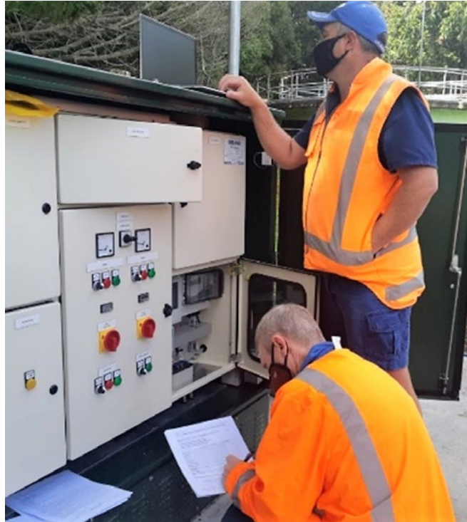
The new wastewater system installed for the residents in Tokanui Village.
