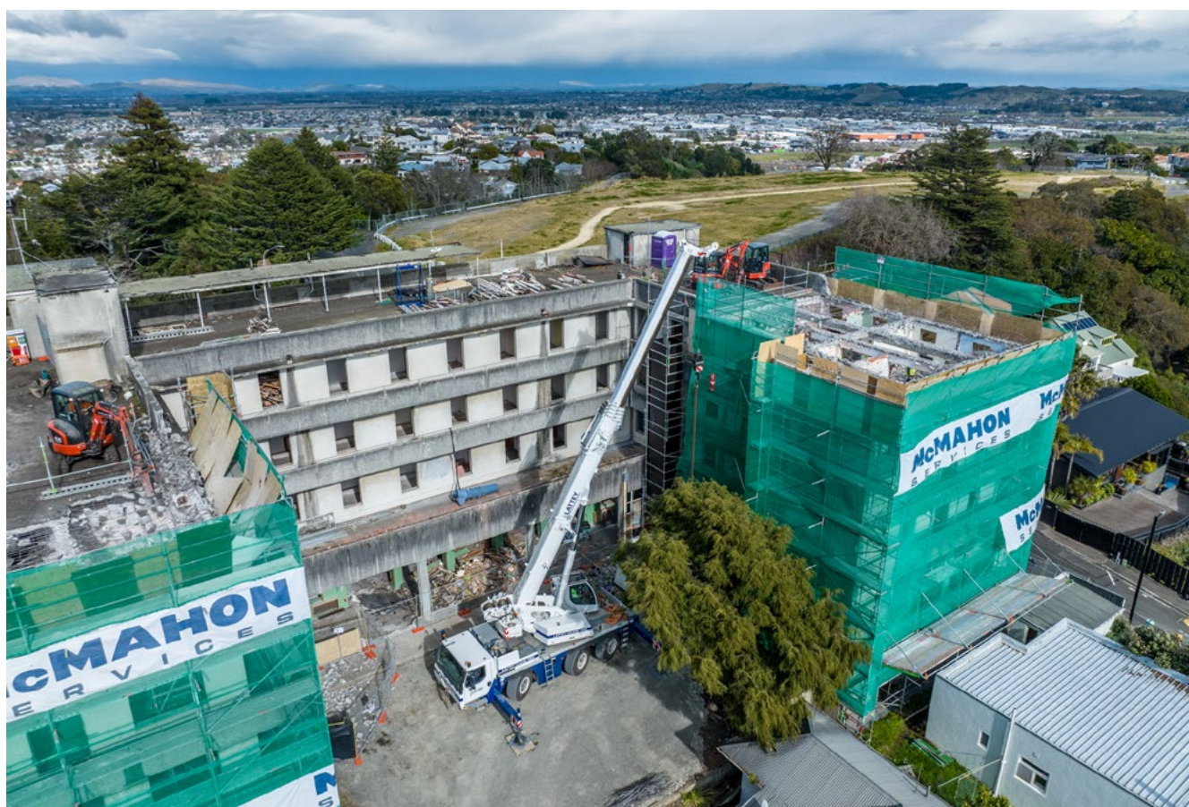
Hinepare Nurses' Home demolition.
