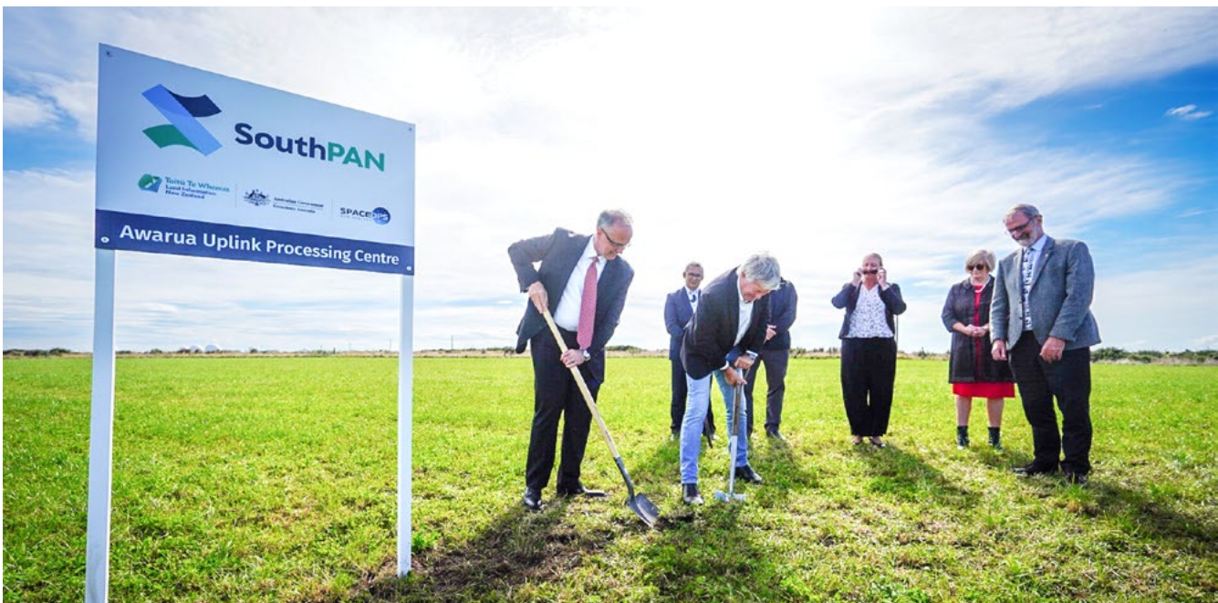
Breaking ground at the Awarua Uplink Processing Centre site. Toitū Te Whenua Kaihautū Jan Pierce, Australian Deputy High Commissioner Amy Guihot, Lockheed Martin Regional Director for Australia and New Zealand David Ball, Land Information Minister Damien O'Connor, Space Ops NZ Ltd CEO Robin McNeill, Te Runaka O Awarua Kaiwhakahaere Dean Whaanga, and Great South Chair Ian Collier.
