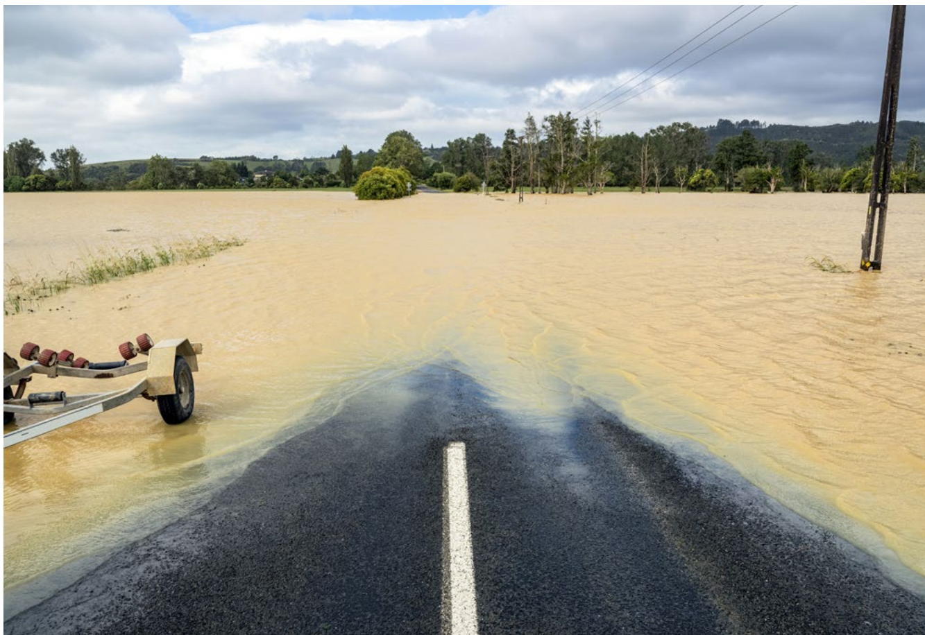
Flooded rural road during Cyclone Gabrielle.
