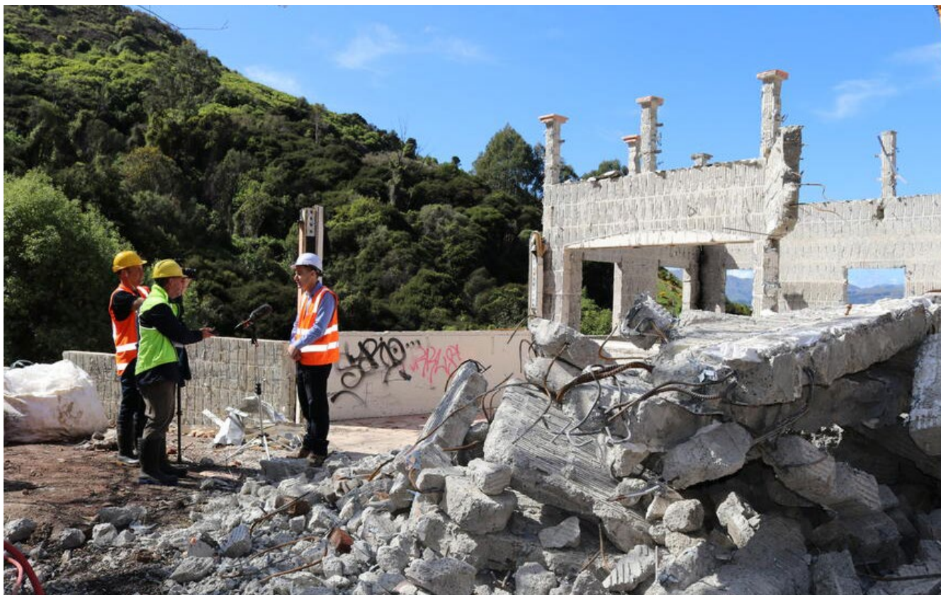
Red zone property in the Port Hills, before demolition started.
