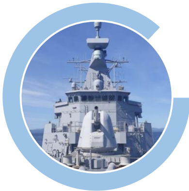
Frigate Sustainment Programme: Phase One
