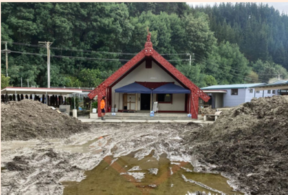
Silt piled high outside Punanga Te Wao at Tangoio Marae following Cyclone Gabrielle. Photo: Heritage New Zealand Pouhere Taonga
