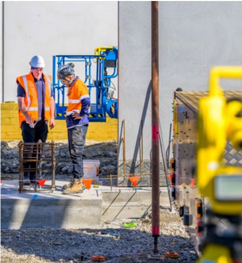
– Springs Road progressing well.
