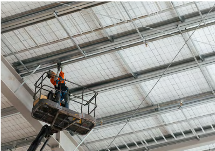
– Roof construction at 30-32 Bowden Road.
