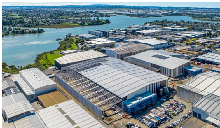
_ Bowden Road construction progress January 2024.
