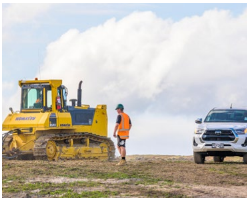
_ Earthworks underway at Spedding Road.
