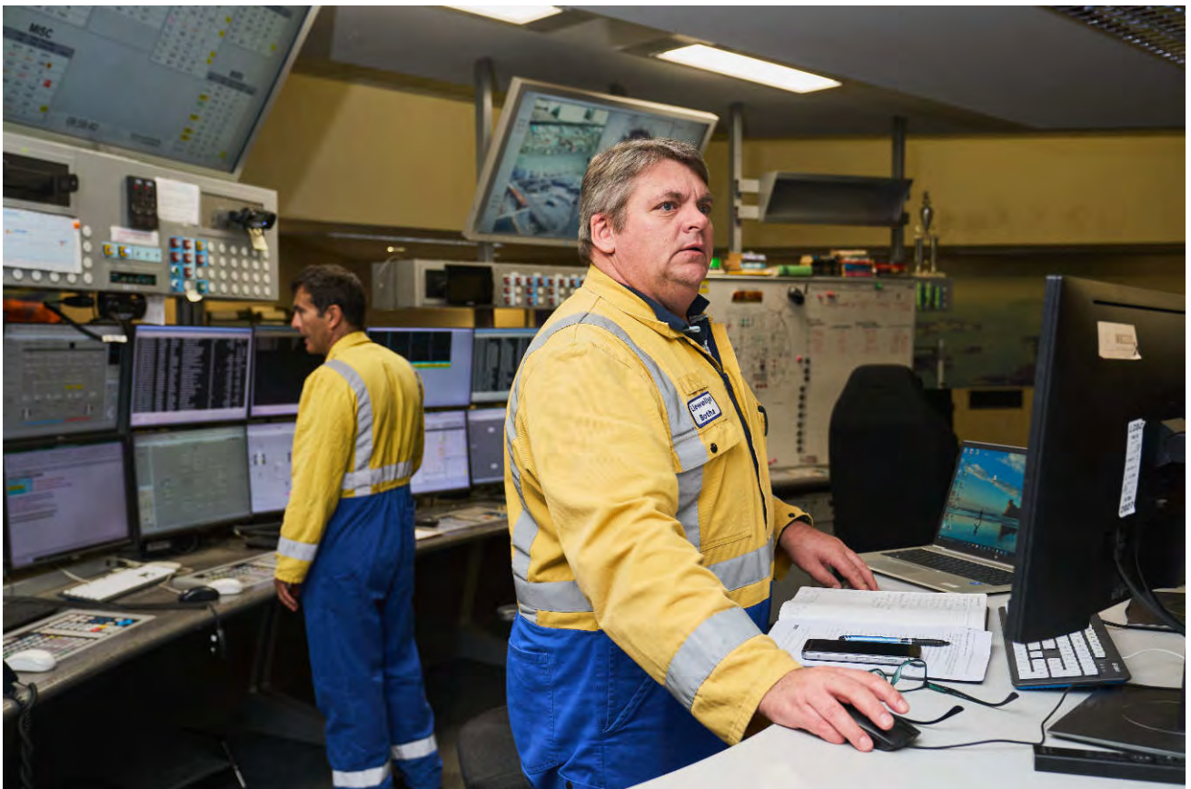
Terminal operators monitoring tank movements and pipeline operations from the control room
