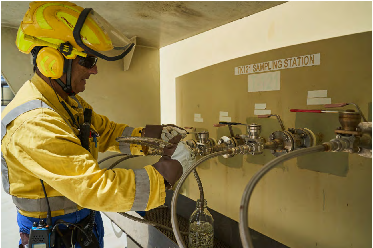
Terminal operator preparing a fuels sample for quality testing by Independent Petroleum Laboratory
