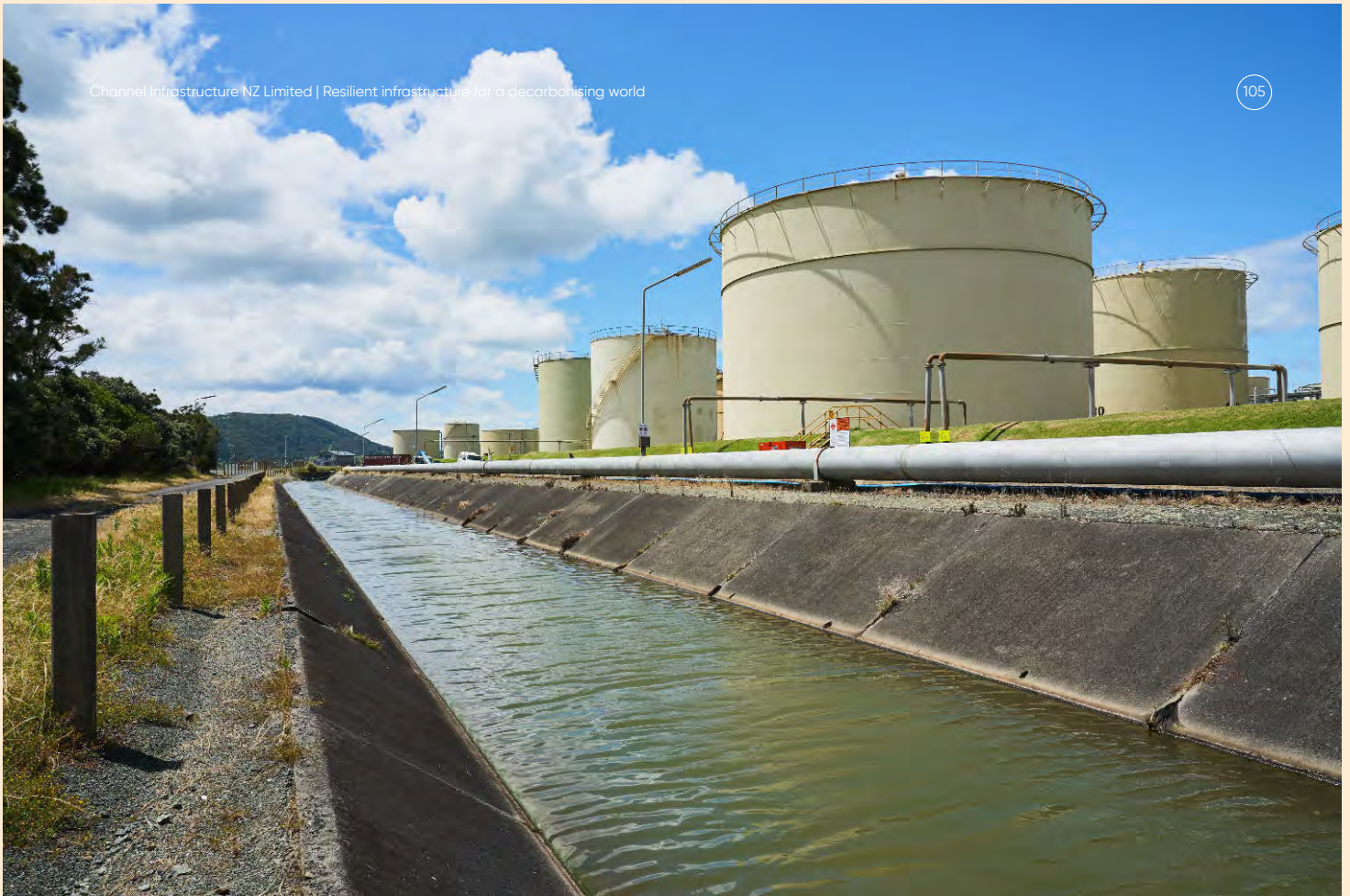
Canals are an integral part of the stormwater network on the Marsden Point site
