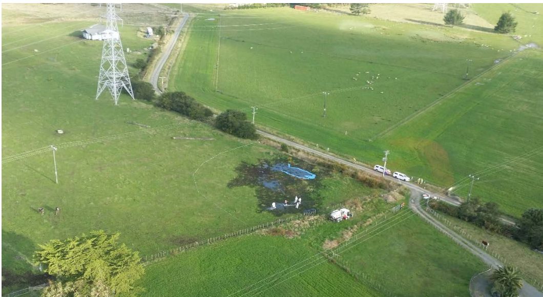
Figure 7: Photograph of the leak site taken from the helicopter, 14 September 2014
